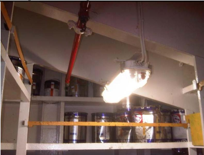
18. Vista de deposito de inflamables a bordo de la draga Marco Polo, completo con sistema contra incendio y lampara antiexplosivas.. / View of the flammable materials storage room aboard the Marco Polo, fitted with fire fighting system and explosion proof lighting.
